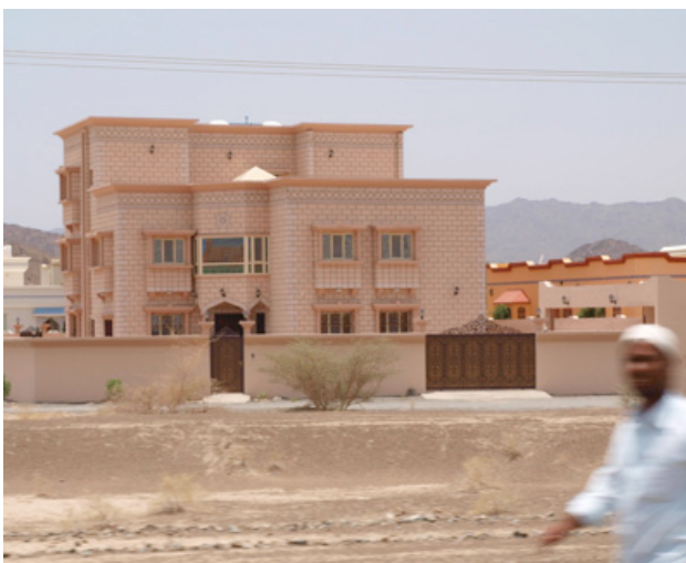
Figure1: The “palace on the plot”, a recent example of urbanization in Muscat Capital Area
