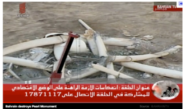
Figure 3: Demolition of Pearl Square
